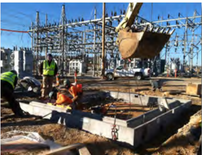
Easy Installation and lightweight sections do not require a crane to set in place
