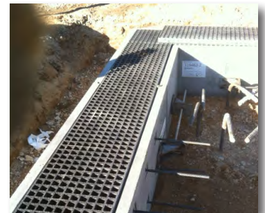
Rounded bottom trench minimizes standing water without the need for sloped floor
